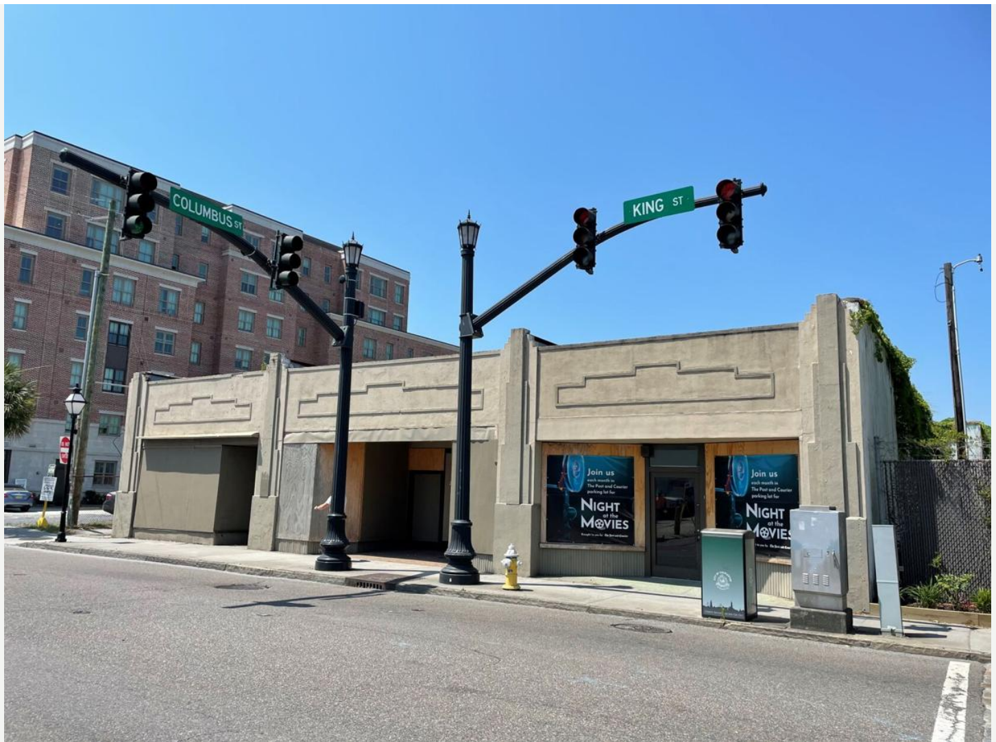
The one-story, early 20th century storefront at 609 King St. Robert Behre/Staff
